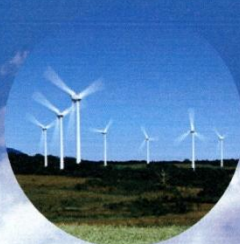
Wind power generation 風力発電
